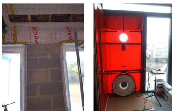
Figure 3: Air Tightness Testing Examples
